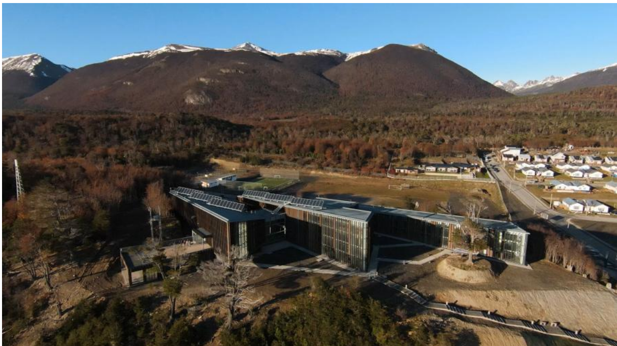
Figure 4. Photograph of the Cape Horn International Center (CHIC) building in Puerto Williams, on Navarino Island, Chile. Photograph by Camilo Quidel, May 2022.
