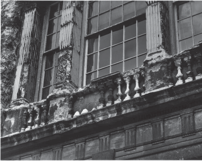
PLATE 1. Badly decayed Headington freestone from Christ Church library, photographed by J.W. Thomas for the Oxford Historic Buildings Fund
