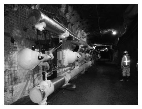
FIGURE 2: Pipes constructed to freeze one of the underground arsenic chambers as part of a Freeze Optimization Study begun in 2009. Photo by Kevin O'Reilly.
