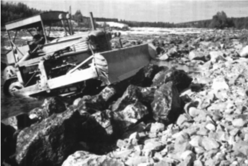
FIGURE 9. Stream-clearing with a Caterpillar, downstream Sågholmen , Degerforsen , in the 1950s.
