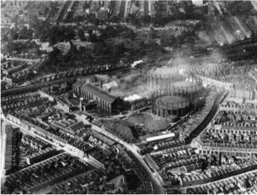
FIGURE 2. Smoke from the Great Central Gasworks drifts over houses in Poplar, Greater London, 1924. 65.3 POP, negative 92/29. Reproduced with permission from London Metropolitan Archives.
