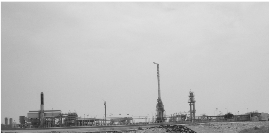
Figure 0.7. Oil refinery at Qasasil, Qatar.
