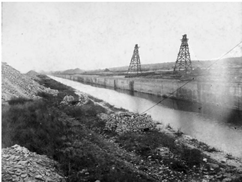
FIGURE 2. Nearly finished Chicago Sanitary and Ship Canal in 1898. Photograph the courtesy of the Lewis University Canal and Regional History Special Collection.
