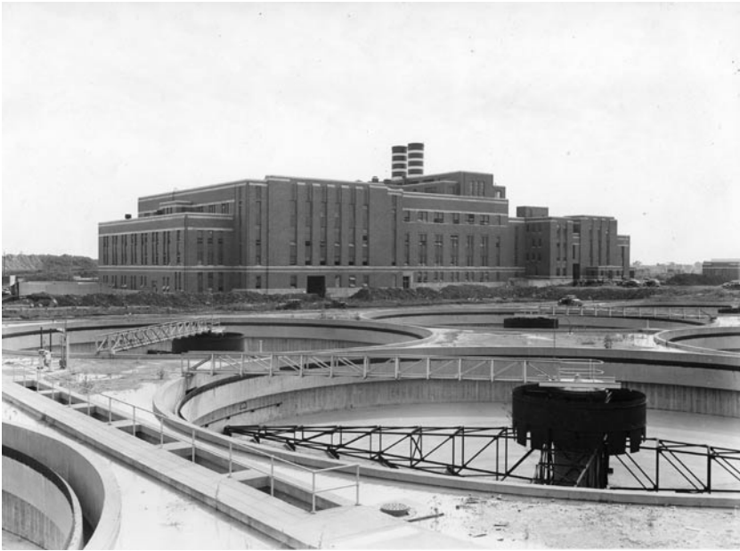
Figure 4. Settling Tanks at the Southwestern Disposal Plant in Chicago which was built as a result of the US Supreme Court's decisions. Photograph the courtesy of the US National Archives and Records Administration (NARA).
