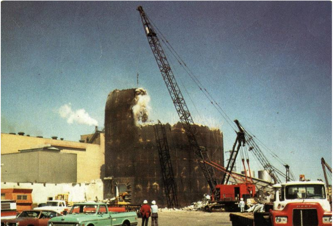
Fig. 5. Decommission job at Elk River, Minnesota, February 1968. Courtesy of US Nuclear Regulatory Commission. Flickr . CC BY-NC-ND 2.0.
