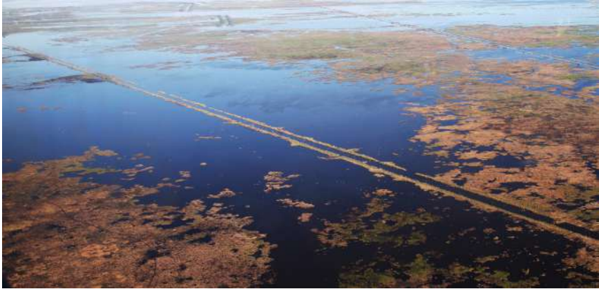
FIGURE 8. Pipeline Canal. Hurricane Ida in 2021 accelerated erosion around this pipeline canal in Lafourche Parish. The estimated 14,000 miles of canals in coastal marsh are major contributors to coastal erosion and subsidence in Louisiana. Photo courtesy of Healthy Gulf c/o Southwings.org.
