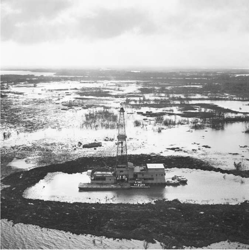
FIGURE 6. Derrick in the Marsh. This undated photo shows an oil derrick surrounded by a waste pit in Terrebonne Parish. A million oil and gas wells have been permitted in Louisiana since the 1901 gusher in Jennings. Oil and gas activities caused more than 70 percent of land loss in the Barataria-Terrebonne basin. Image courtesy of the Historic New Orleans Collection, © Douglas Baz and Charles H. Traub, 2019.0362.93.
