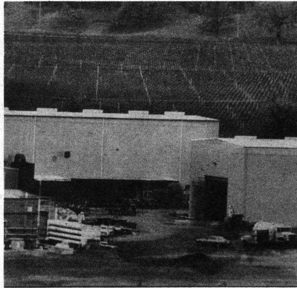
The Retech Facility South of Ukiah
