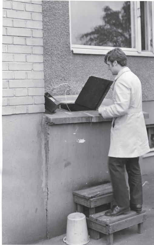
Pic 3. Health inspector Pauli Lindfors measuring the combustion temperature of a backyard incinerator in Helsinki in the 1960s 52
