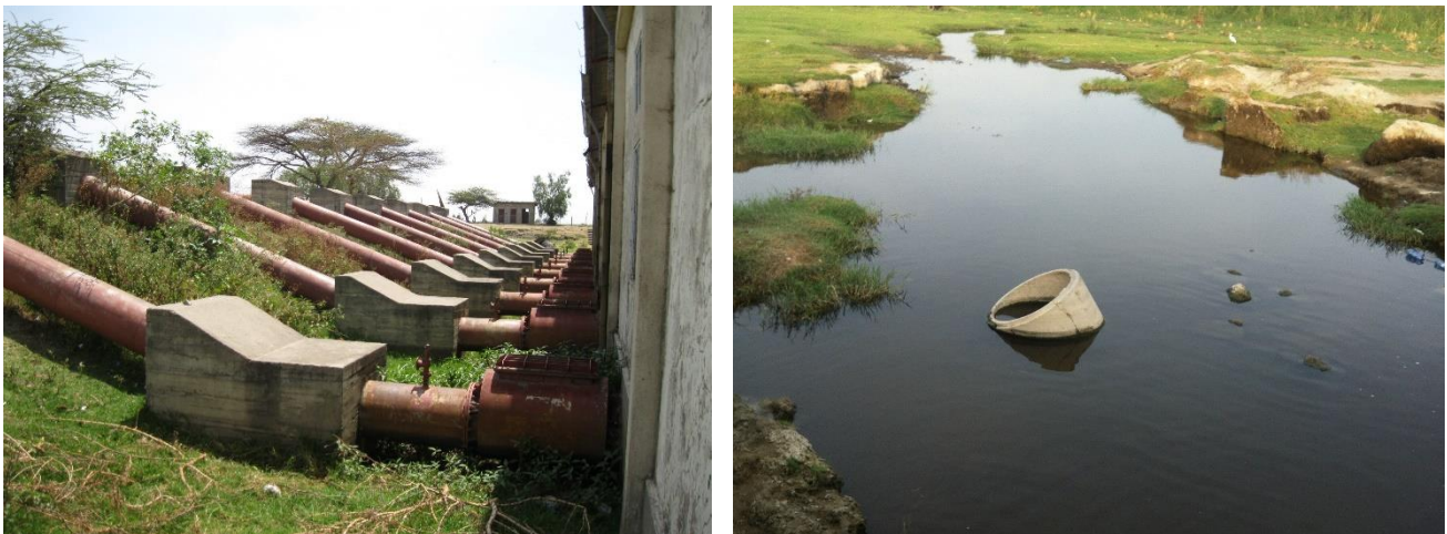
Fig. 7 and 8: Electric pumps to remove water from the lake and wastewater discharge to Lake Ziway from floriculture industries. © Hayal Desta. All rights reserved.
