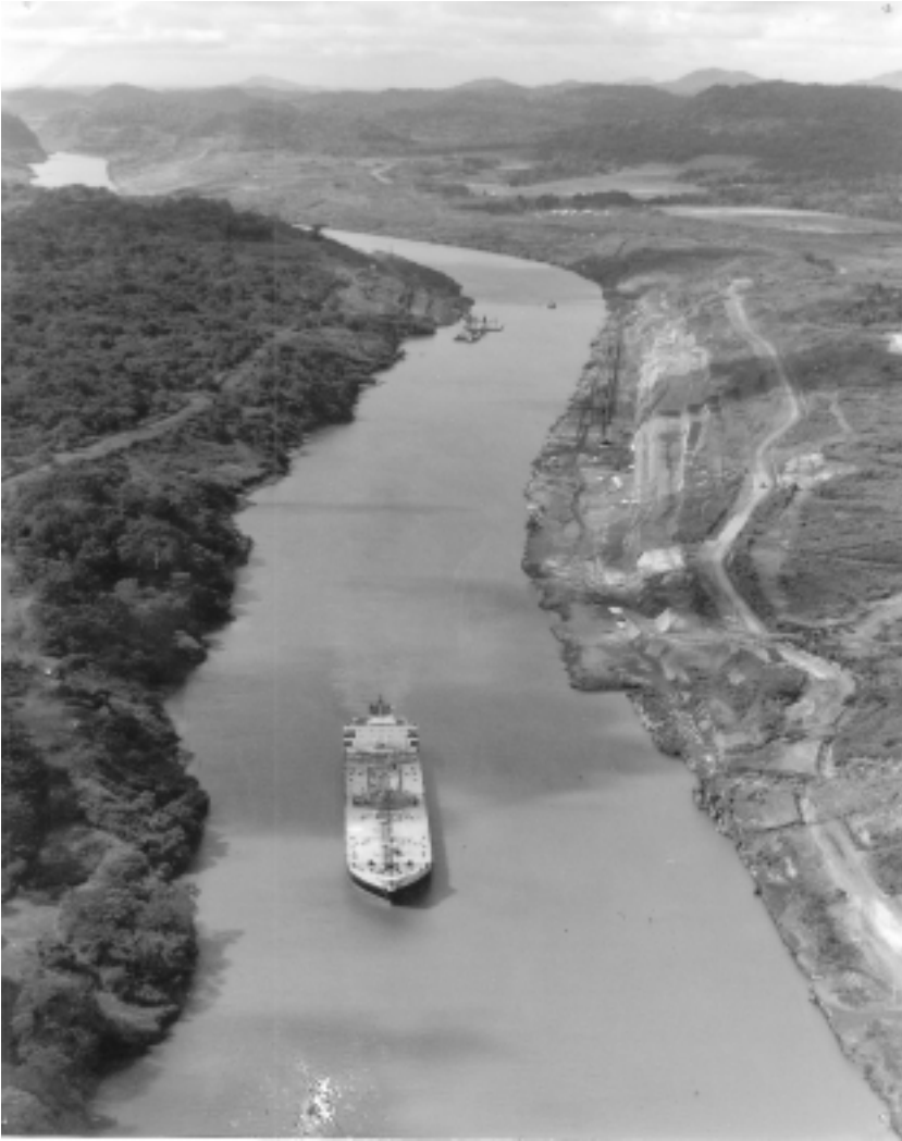
FIGURE 4. The Gaillard (formerly Culebra) Cut, from which 115 million cubic yards were excavated during construction
