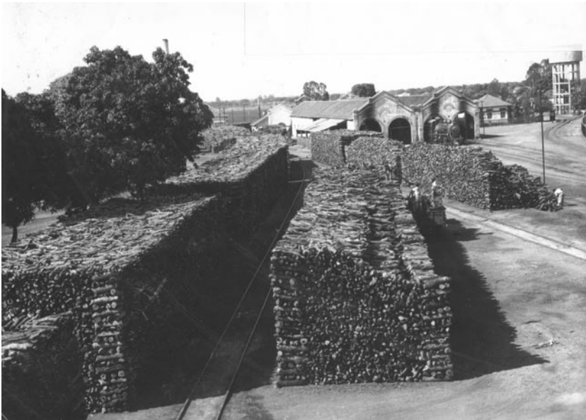
FIGURE 7. Fuel wood for Noroeste railroad locomotives, c 1940, Tres Lagoas, Mato Grosso state (presently Mato Grosso do Sul). Source: Helder Barros, 'Noroeste' (1989), Centro de Memória Regional, UNESP-RFFSA, Bauru.
