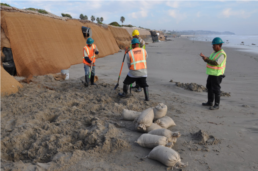
Building a flood protection wall at Broad Beach, Malibu.
