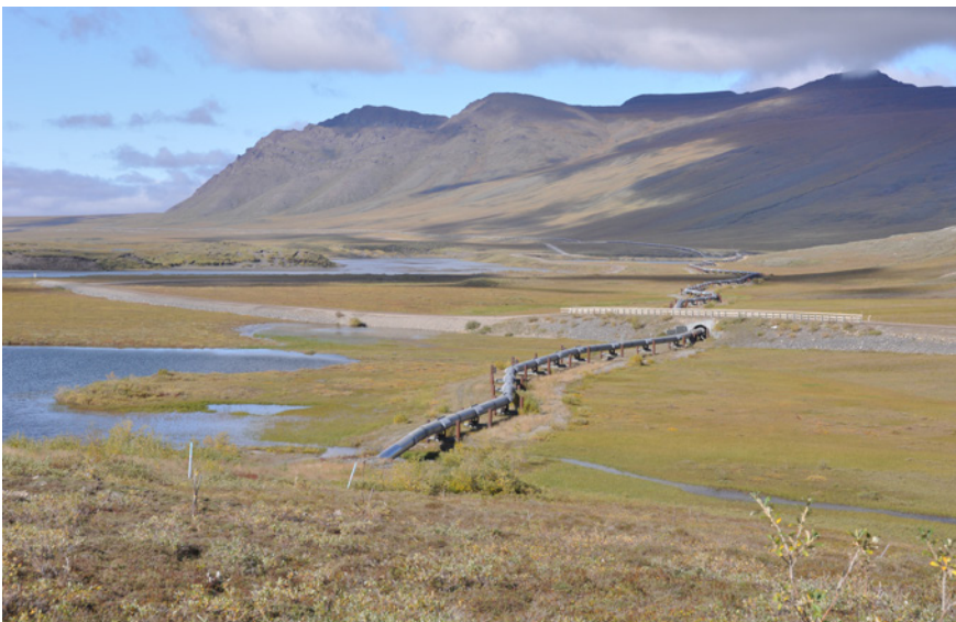
Dalton Highway and oil pipeline, north of the Gates of the Arctic National Park.
