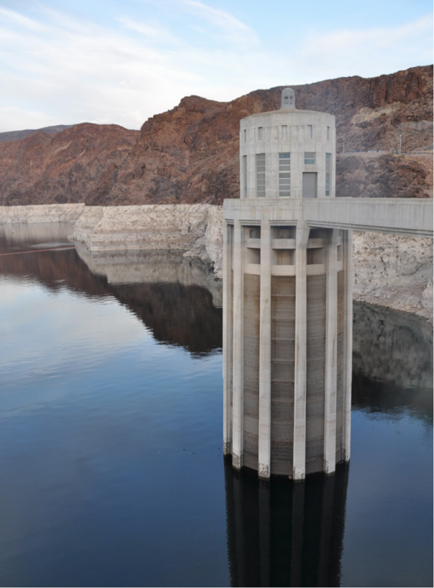
A white 'bathtub ring' at Hoover Dam has bleached the rocks of Lake Mead. It shows how the water level has dropped over the last decades.
