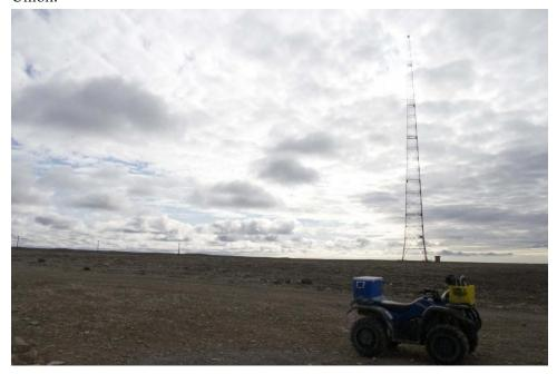
No. 28. The Cambridge Bay long-range navigation (LORAN) tower was built in 1947–48 for radio transmissions. It was 189 meters tall and was used until recently as a non-directional beacon. The tower was demolished in August 2014 because it was structurally unsound. Cambridge Bay, Nunavut. August 2013. Photos taken by Enrico Mariotti.
