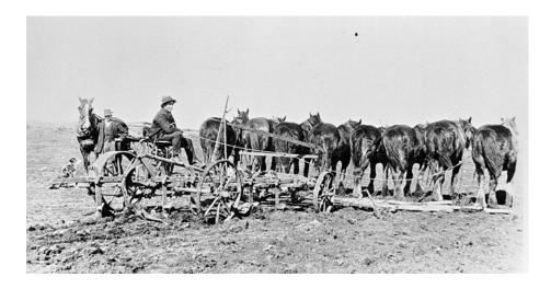
Figure 4: Ploughing with a stump-jump plough
