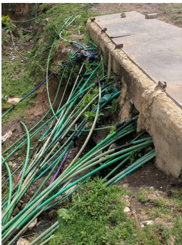
A “chamber”: a locked concrete box with legal metered connections to the grid, Kibera 2021.
