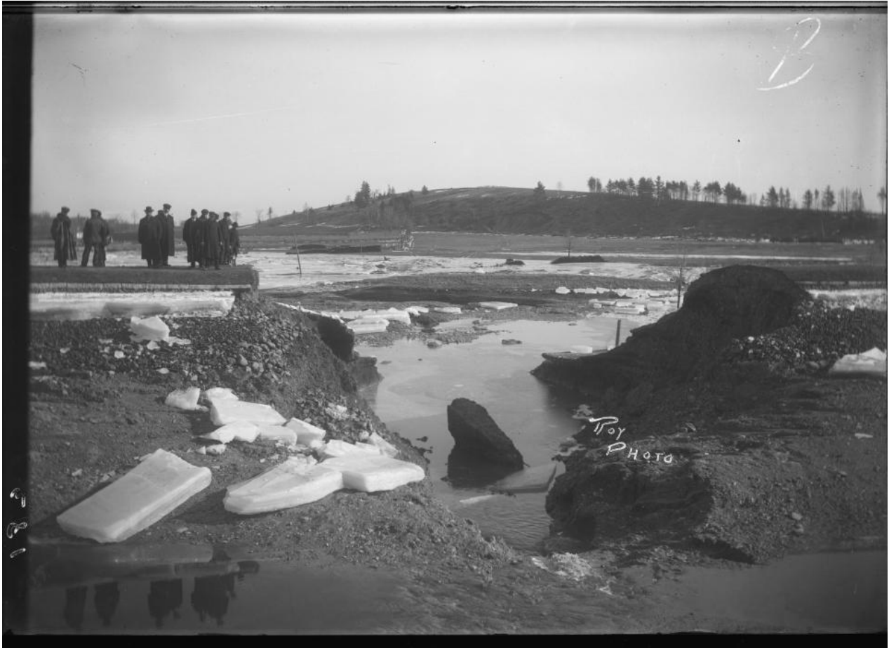
Aftermath and damage of canal break above Peterborough Lift Lock.
