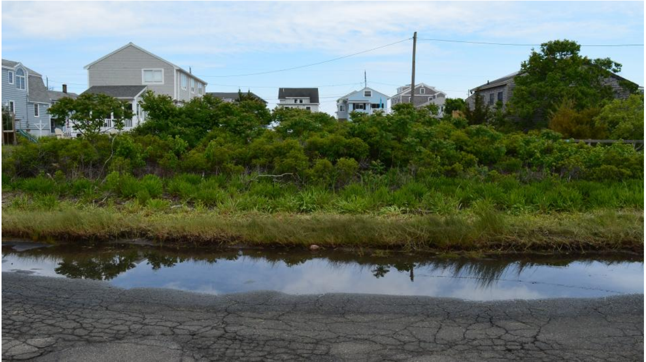
Sunny day flooding at mid-tide on Long Beach Road, the privately owned access road to the cottages. The road is one example of an impervious surface on Long Beach that limits water from percolating into the soil.
