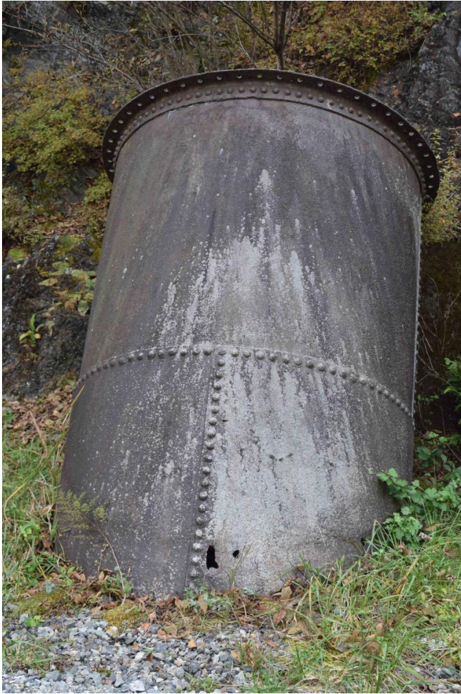
Some of the ruins of the Matō Hydroelectric Power Plant. The photo shows remnants of piping through which water fell 31.8 meters to power the turbine.
