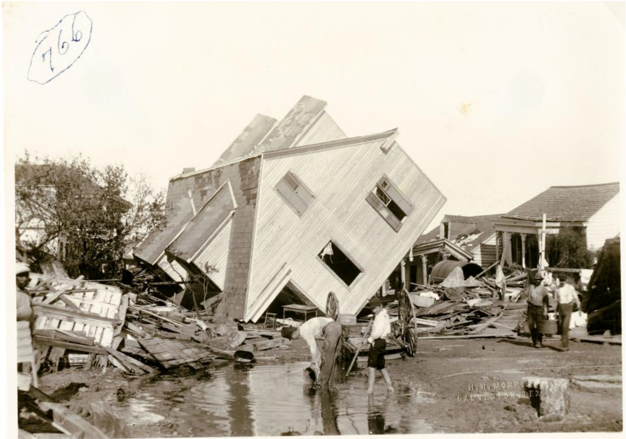
Men working near an overturned house after the Great Storm.
