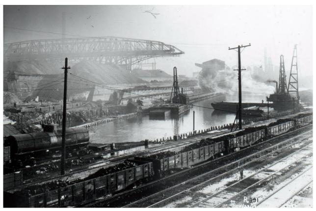
South Slip at South Works, 1917. This artificial inlet received ore and coal to be distributed by rail cars within the steel plants. Note the coal mountain within the ore walls just beneath the gantry cranes. Courtesy of the Southeast Chicago Historical Society [Archive ID: 1983-100-d22]. All rights reserved.
