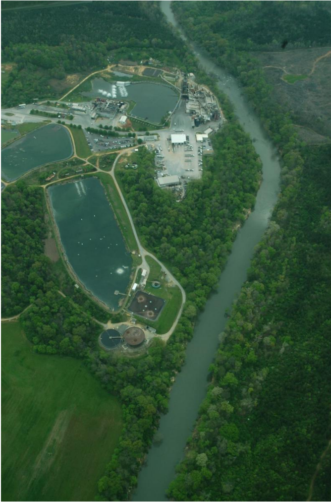
Aerial photograph of the Tyson Rendering Plant in Hanceville, Alabama.
