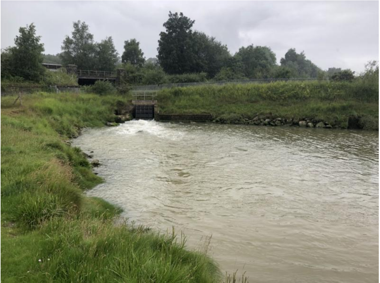
The outfall channel of the Milwr Tunnel near Bagillt on the Dee Estuary is known locally as “The Holy.”
