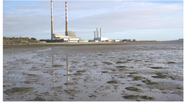
Ringsend's generating station in 2017. The Poolbeg chimneys are colloquially known as the "Poolbeg stacks."
