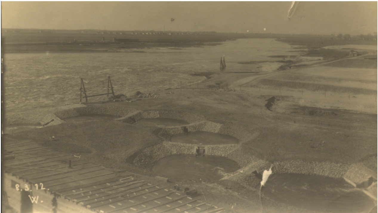
The bypass channel ( Wildpass ) at the Hemelinger Dam with its extensive and light-filled basins—a design that bears Landmark’s signature.
