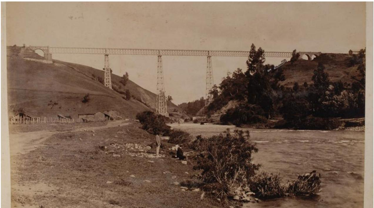
The Malleco Viaduct in 1890, with a length of 408 meters and a height of 102 meters.
