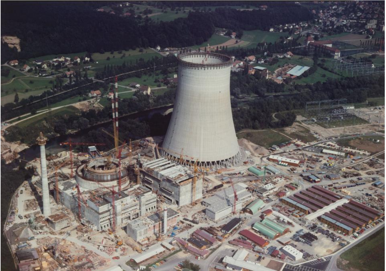
The construction of Gösgen Nuclear Power Plant in 1976.
