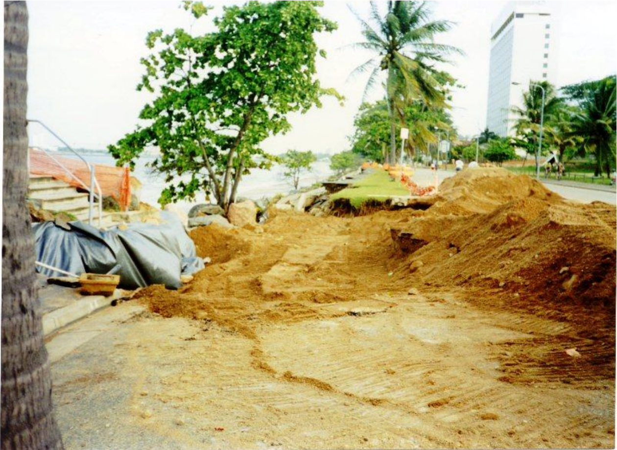
Photograph showing damage to Townsville's Strand, 15 January 1998.
