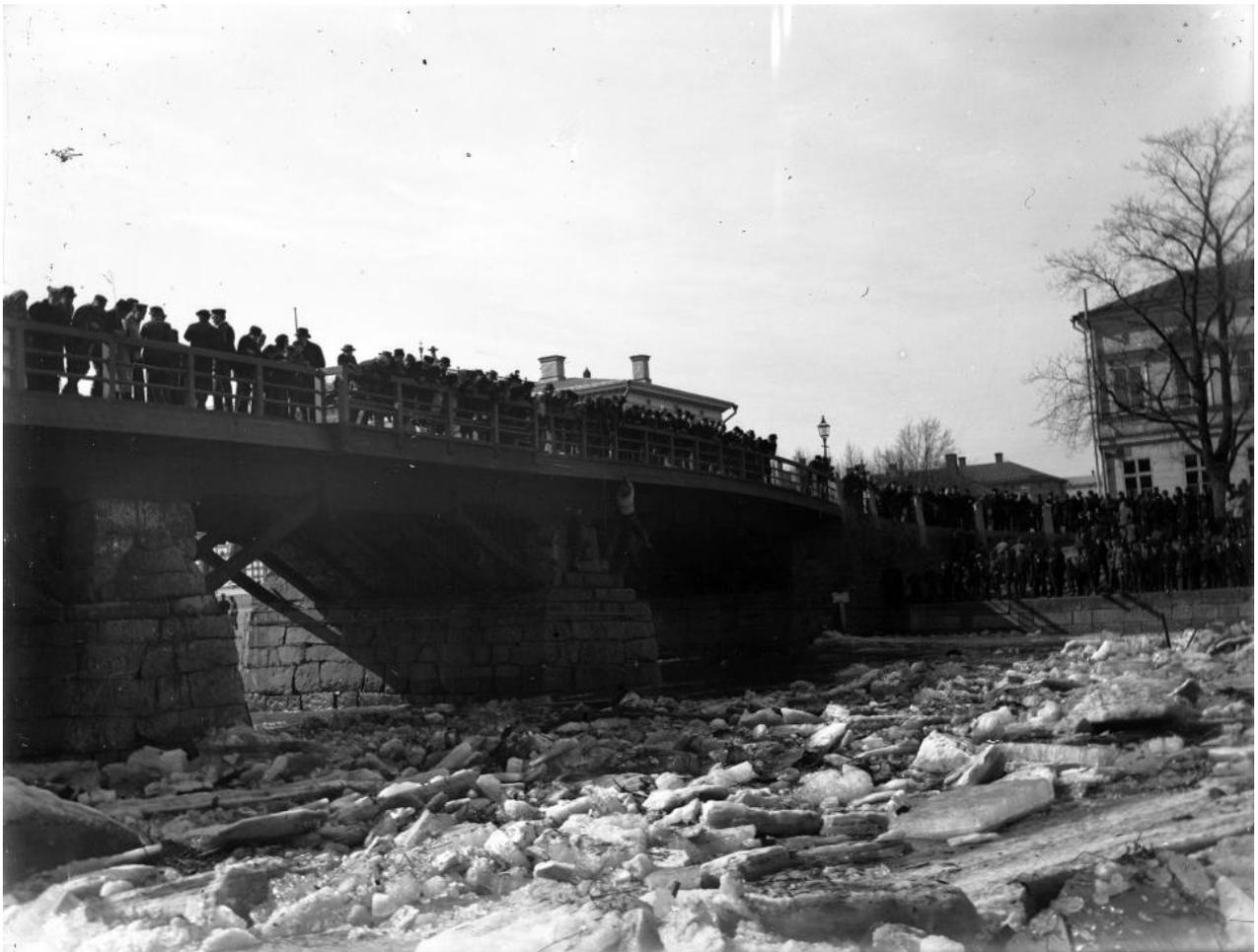
Ice jams usually occurred in front of Aura Bridge. This photo from 1897 shows the belt of steel that was attached to one of the pillars (the pillar further away from the camera) to hinder it from falling down.
