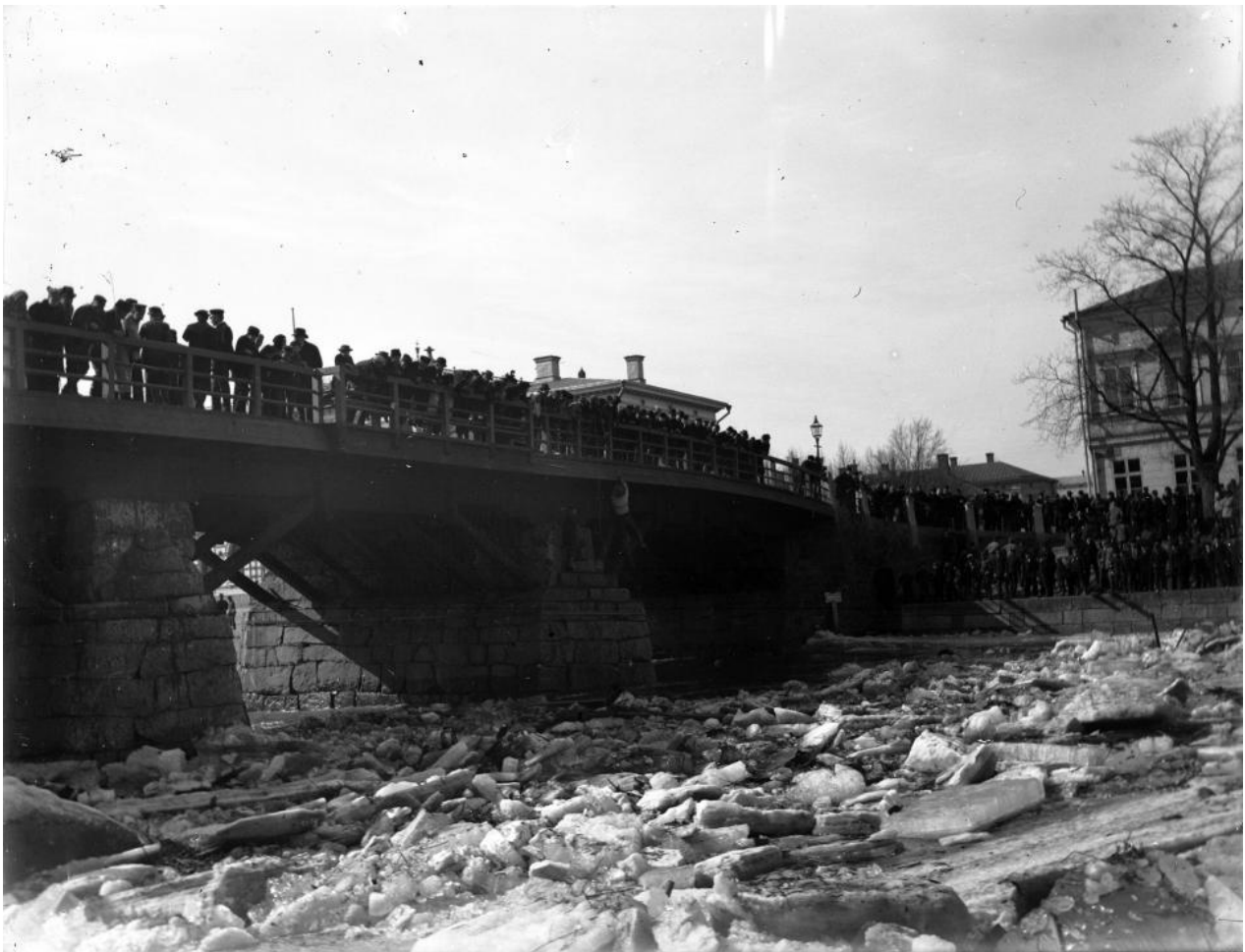
Ice jams usually occurred in front of Aura Bridge. This photo from 1897 shows the belt of steel that was attached to one of the pillars (the pillar further away from the camera) to hinder it from falling down.
