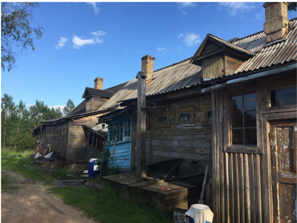
Figure 2. Houses in Workers' Settlement no. 13.
