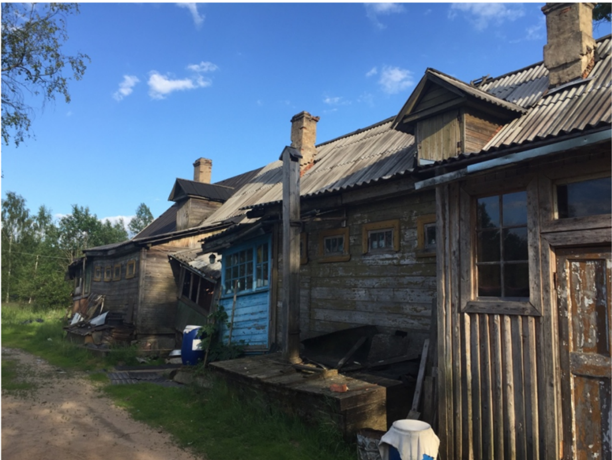
Figure 2. Houses in Workers' Settlement no. 13.
