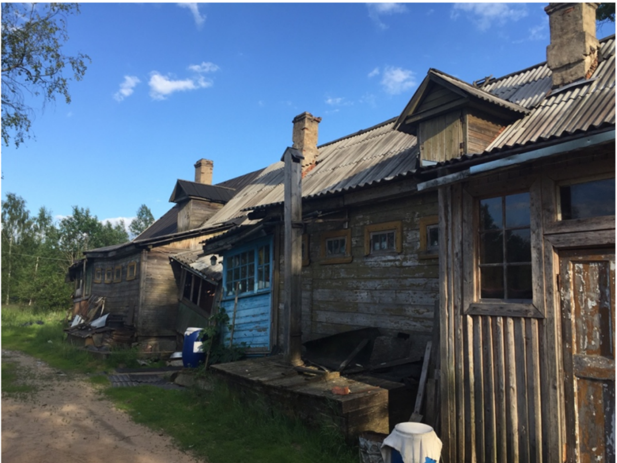
Figure 2. Houses in Workers' Settlement no. 13.
