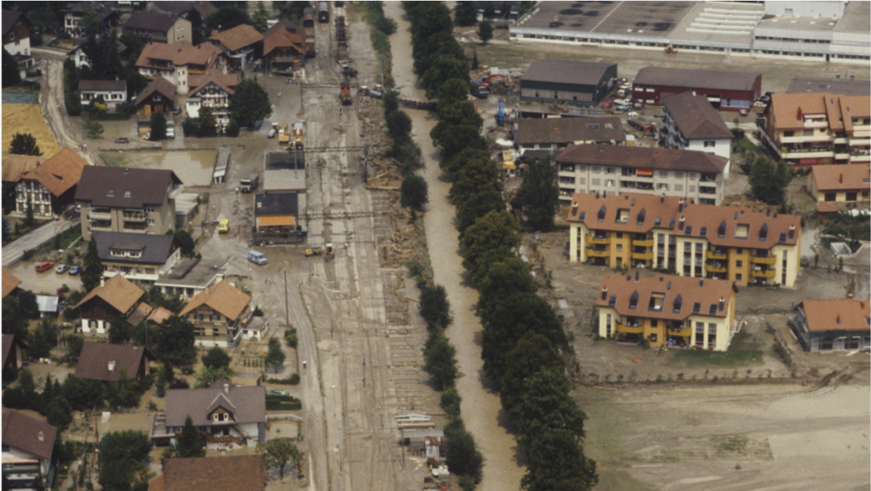
Flooded settlement in Toffen after the event of 29 July 1990.
