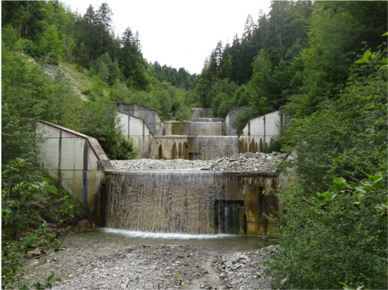
Torrent check dams in the gorge of the Gürbe River.
