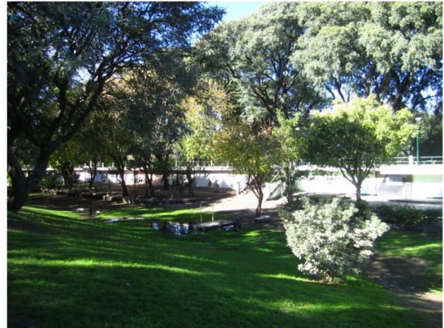
Present-day view of the breakwater from the same location, June 2014. The breakwater has been renovated and reopened to the public recently.
