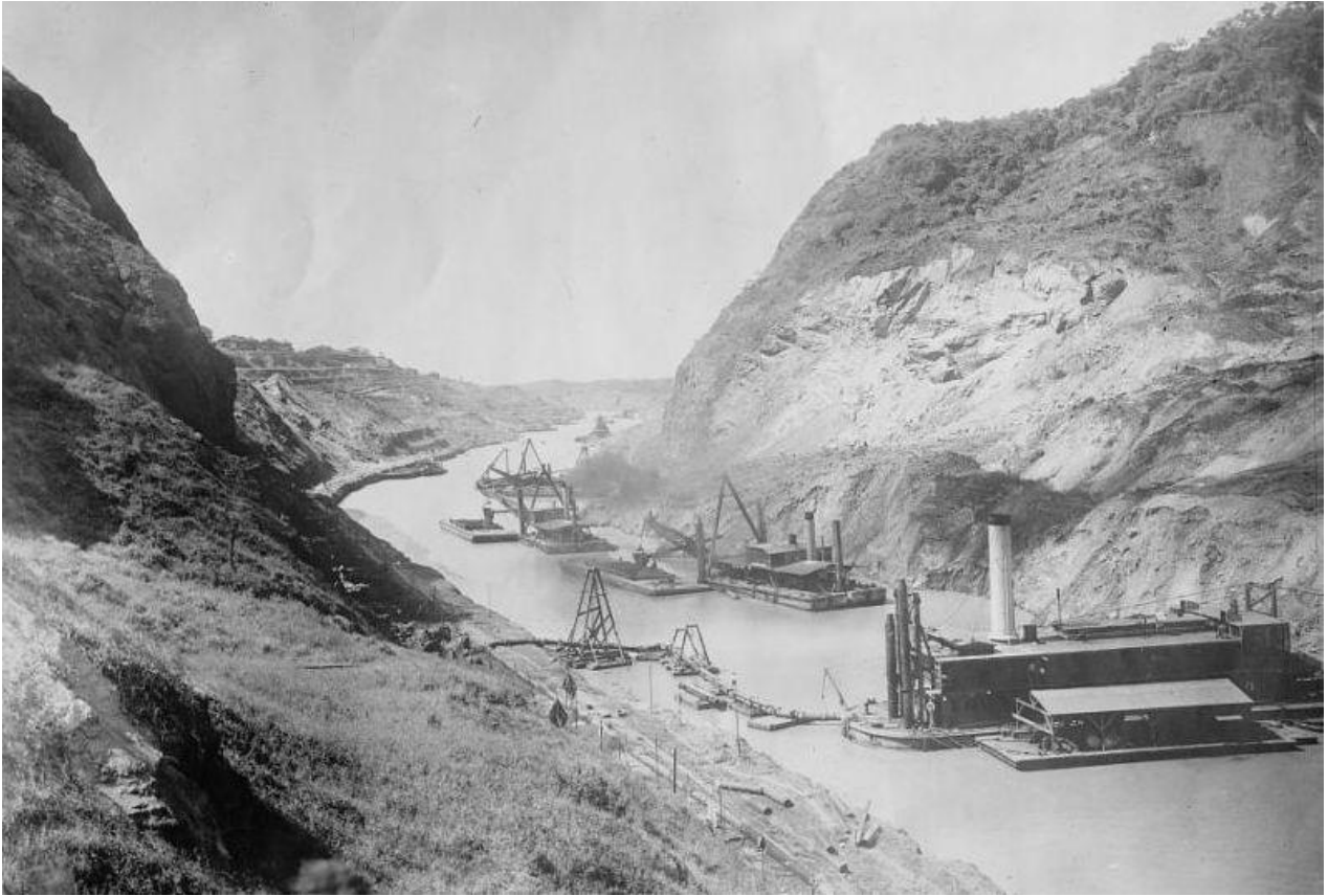
Photo of the dredges removing material from the Cucaracha slide in the Culebra Cut, ca. 1913.
