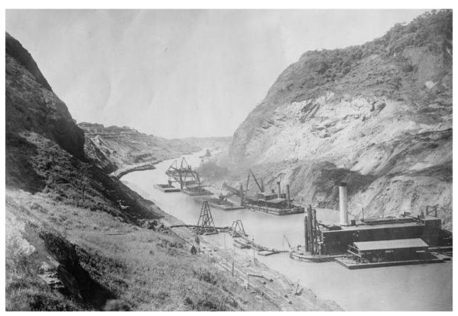
Photo of the dredges removing material from the Cucaracha slide in the Culebra Cut, ca. 1913.
