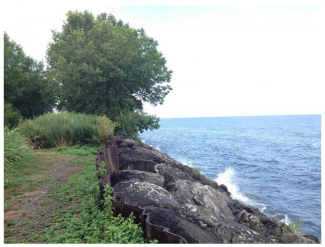
The Army Corps created containment areas using techniques developed to make land for other purposes: driving steel into the lakebed and protecting it with stone. Although the process removed habitat from the lake, proponents argued that the rocks would provide new habitat for aquatic species.
