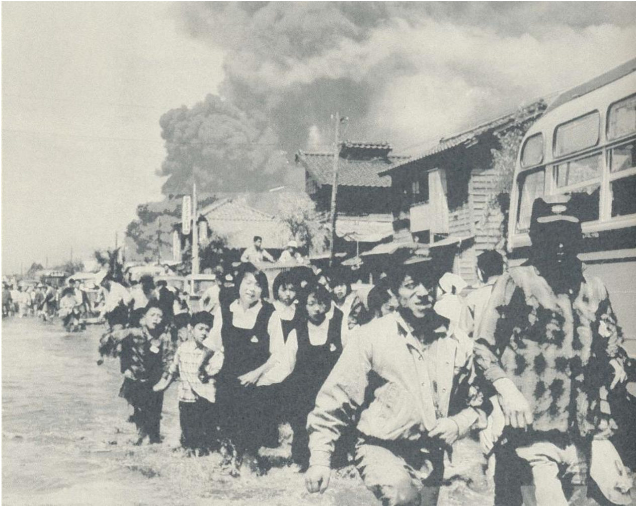
Tsunami-inundated Niigata City, 1964. This image was provided by Niigata Nippo Sha .
