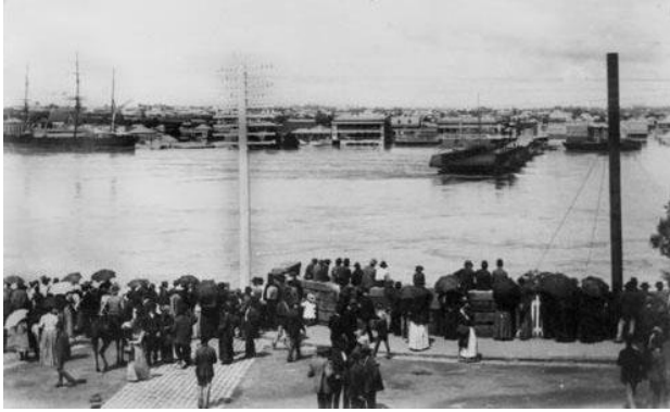
Victoria Bridge, connecting north and south Brisbane, destroyed by floods
