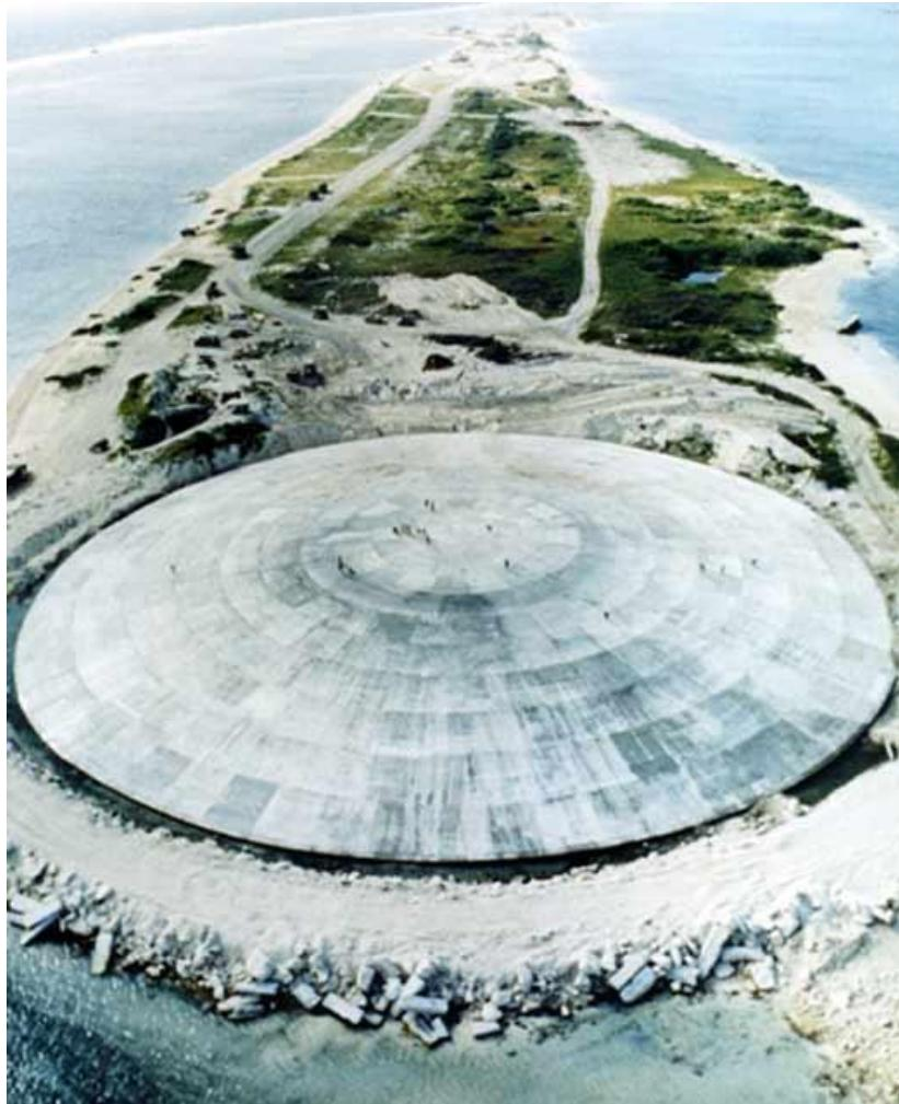
Dome on Runit Island, Enewetak Atoll, Marshall Islands, covering a crater created by a US nuclear weapons test in 1977. The crater and dome now contain 84,000 cubic meters of radioactive soil from other islands in the Enewetak Atoll. Unknown photographer.
