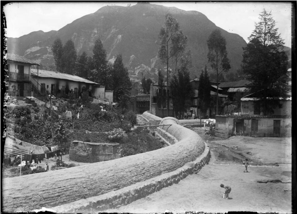
Canal río San Francisco (Photographed by Acuña, Luis Alberto [1930]). San Francisco River Channel, 1930.
