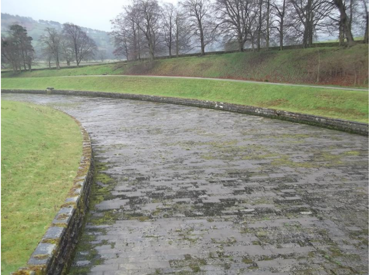
The dry by-wash at Swinsty, which allows water to flow down the valley to Lindley Wood Reservoir by means of gravitation.
