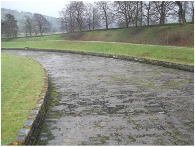
The dry by-wash at Swinsty, which allows water to flow down the valley to Lindley Wood Reservoir by means of gravitation. Photo taken by Andrew McTominey, 2016.
