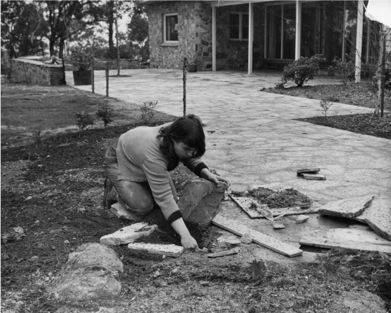
Margot Knox doing some paving (1960s)
