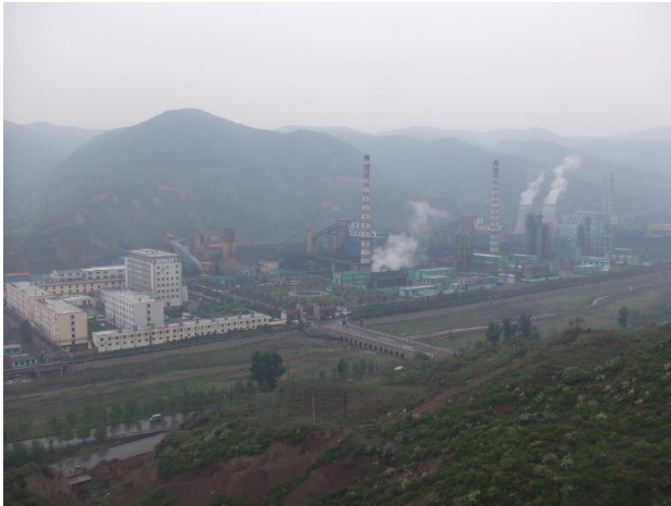
View of four cokeries in the Gujiao area with an annual capacity of 3.8 million metric tons per year before their integration into a combined coke processing facility
