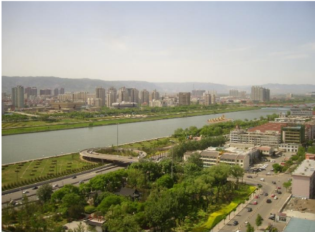
Northbound view of Fen River Park near Yingze Street, Taiyuan, Shanxi Province, China
