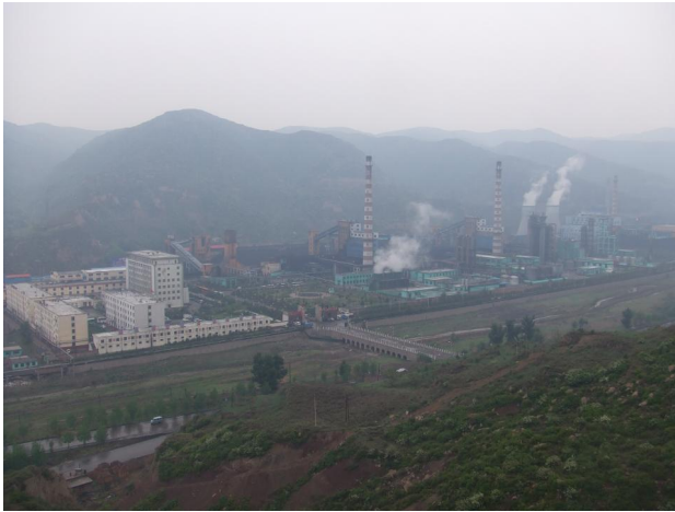
View of four cokeries in the Gujiao area with an annual capacity of 3.8 million metric tons per year before their integration into a combined coke processing facility
