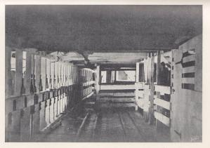
Fig. 16.-Main deck of horse-carrying three-decker, showing stalls at starboard side and midship stalls.
