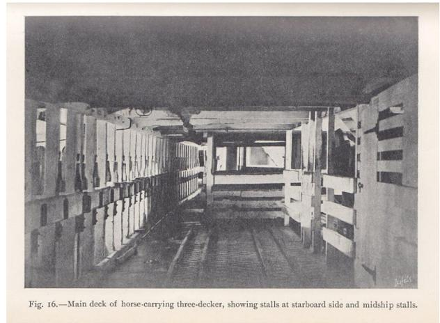
Fig. 16.—Main deck of horse-carrying three-decker, showing stalls at starboard side and midship stalls.
