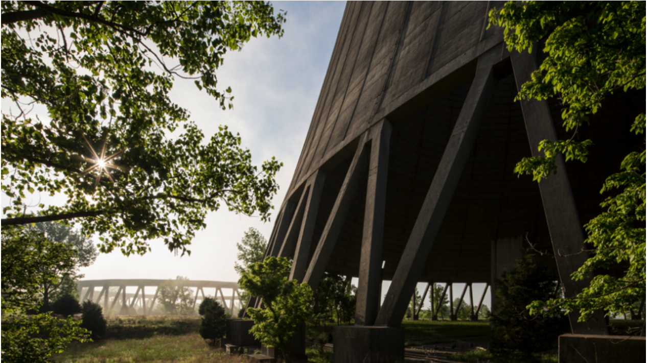
Hartsville's cooling tower
