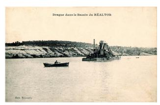
Barge-mounted hydraulic dredge operating at the surface of a storage and sedimentation reservoir originally built along the Canal de Marseille: the Réaltor reservoir (early twentieth century)
