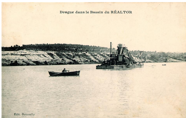
Barge-mounted hydraulic dredge operating at the surface of a storage and sedimentation reservoir originally built along the Canal de Marseille: the Réaltor reservoir (early twentieth century)
