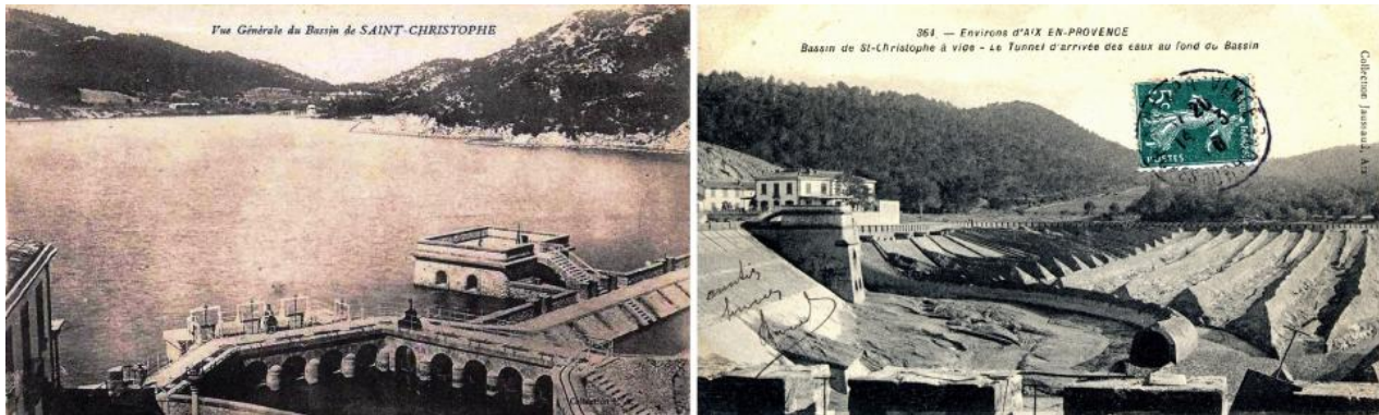
The Saint Christophe reservoir: full of water and operational (left photo) and empty during a desilting campaign (right photo). Both postcards are from the early twentieth century.
