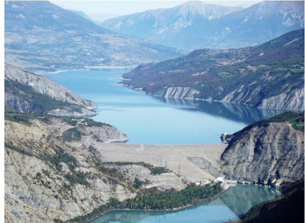
The Serre-Ponçon dam and the lake in 2013 (looking upstream from the left bank)
