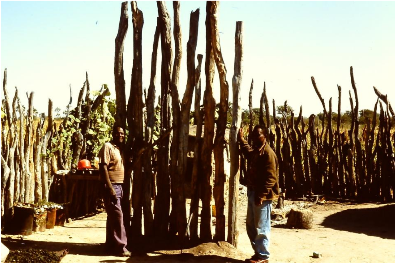
View of the inside of a palisaded homestead in 1992. The palisade poles between the two men are recycled poles from the palisade surrounding the original homestead which was constructed in the 1920s, when the threat of wild animals was still real. Today's palisade, which is seen in the background, is much lower, reflecting the fact that when it was built during the 1980s, poles were increasingly scarce and predators were no longer a threat to this village.
