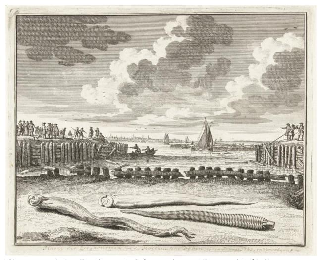
This contemporary print shows dike workers removing piles from a coastal revetment. The exaggerated size of the shipworms was a pictorial convention, but it also accentuated the monstrous interpretation of this invasive species.
