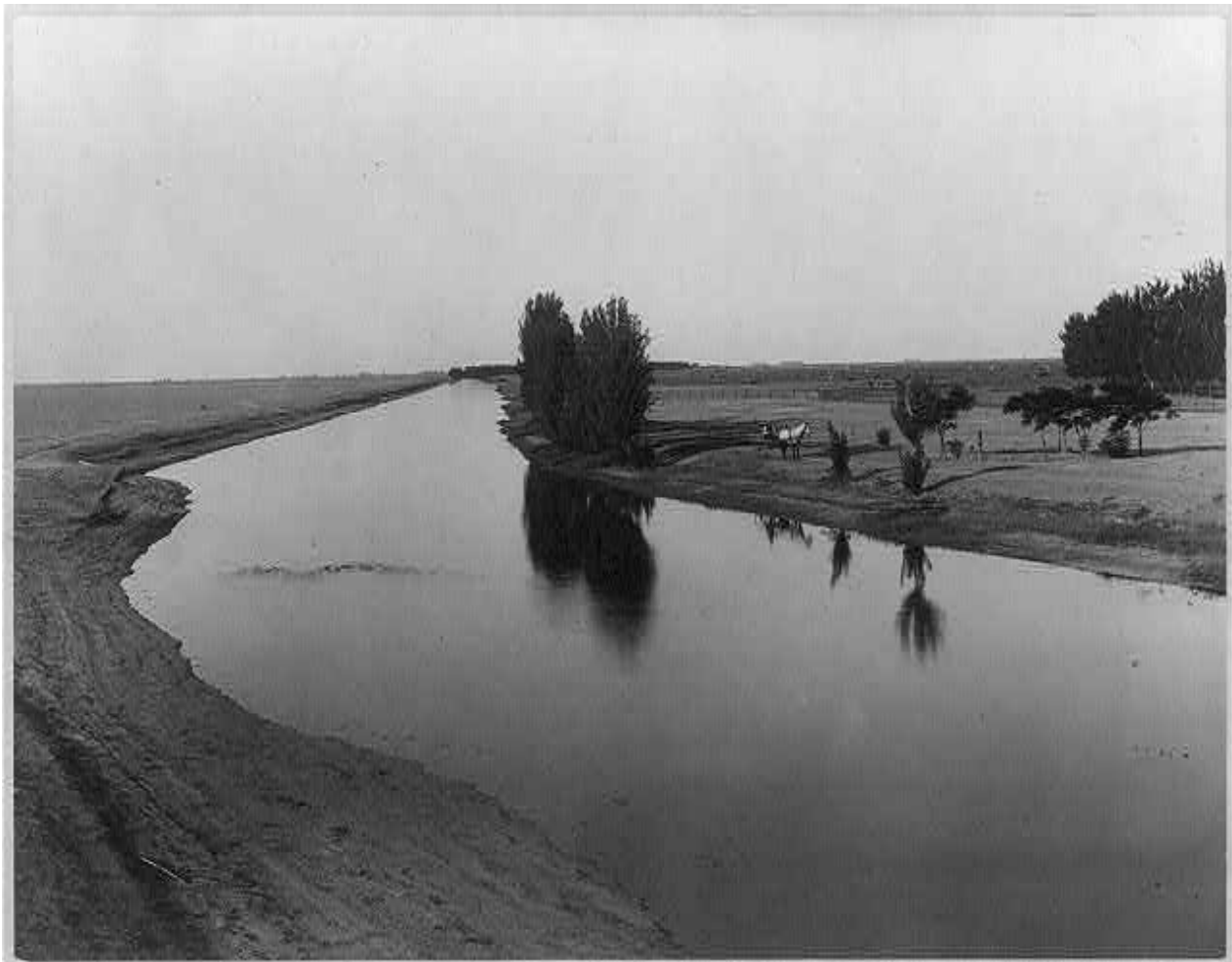
The Calloway Canal near the headquarters of the Poso Ranch in Kern County, California.
